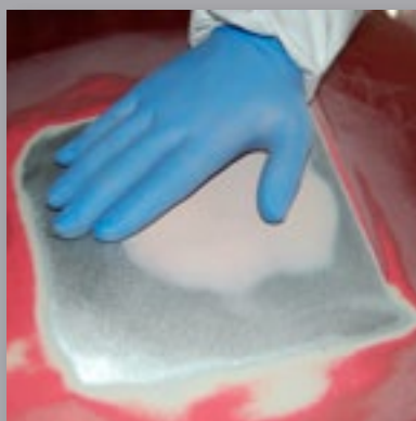
8 Final inspection ready for primer application process.
